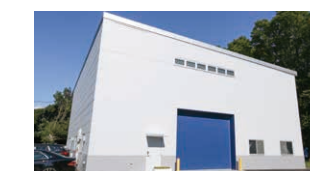
The sound insulation testing lab
