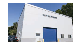
The sound insulation testing lab
